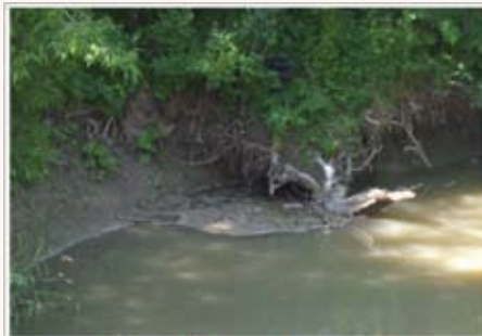
Vertical bank with exposed soil
